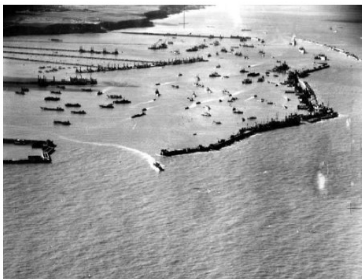
The Mulberry Harbour built during the days following D-Day at Arromanches in Northern France, to get troops and vehicles off the ships and onto shore as fast as possible. To the right is the 'harbour wall' - around 100 old ships sailed across the Channel and scuttled. Within the harbour can be seen the Phoenix Caissons, floating concrete piers (one of which can still be seen off Thorpe Bay), and the Spud Piers, long pontoons which connected to the land. All of this was part of the huge transport effort mounted, starting on D-Day, and still the largest seaborne invasion in history.
